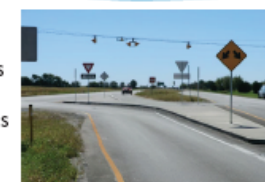
Example of RCUT Intersection. Source: FHWA
