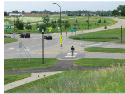
Example of a multi-lane roundabout.
